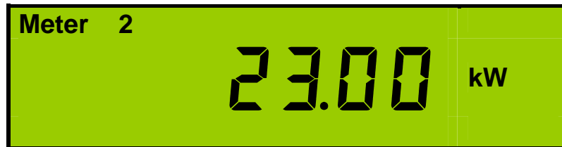
Active Power - Meter 2
